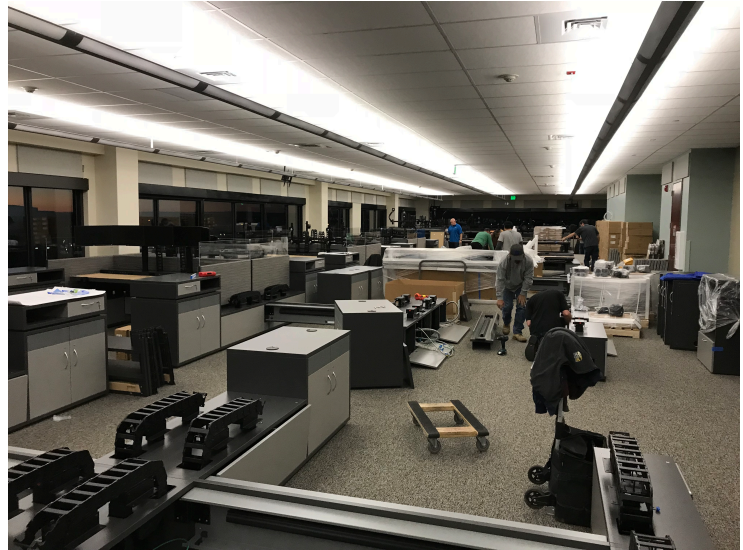
Construction of Communications Floor (2017)
